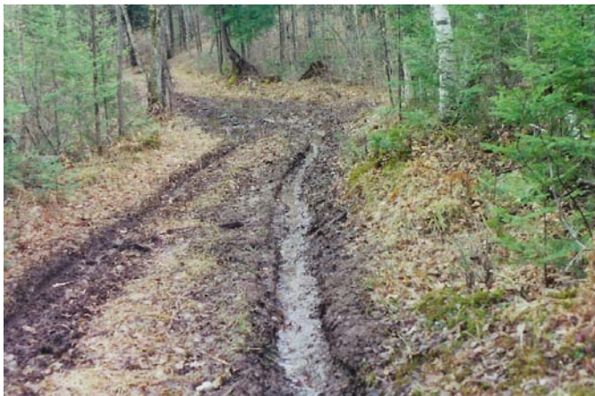
Damage to 566A by 4 wheel drive vehicles.
